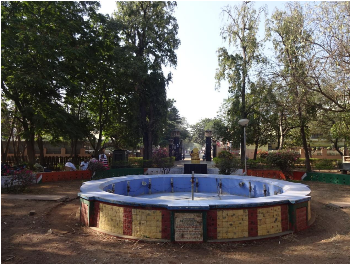
Existing Condition of Water Fountain
