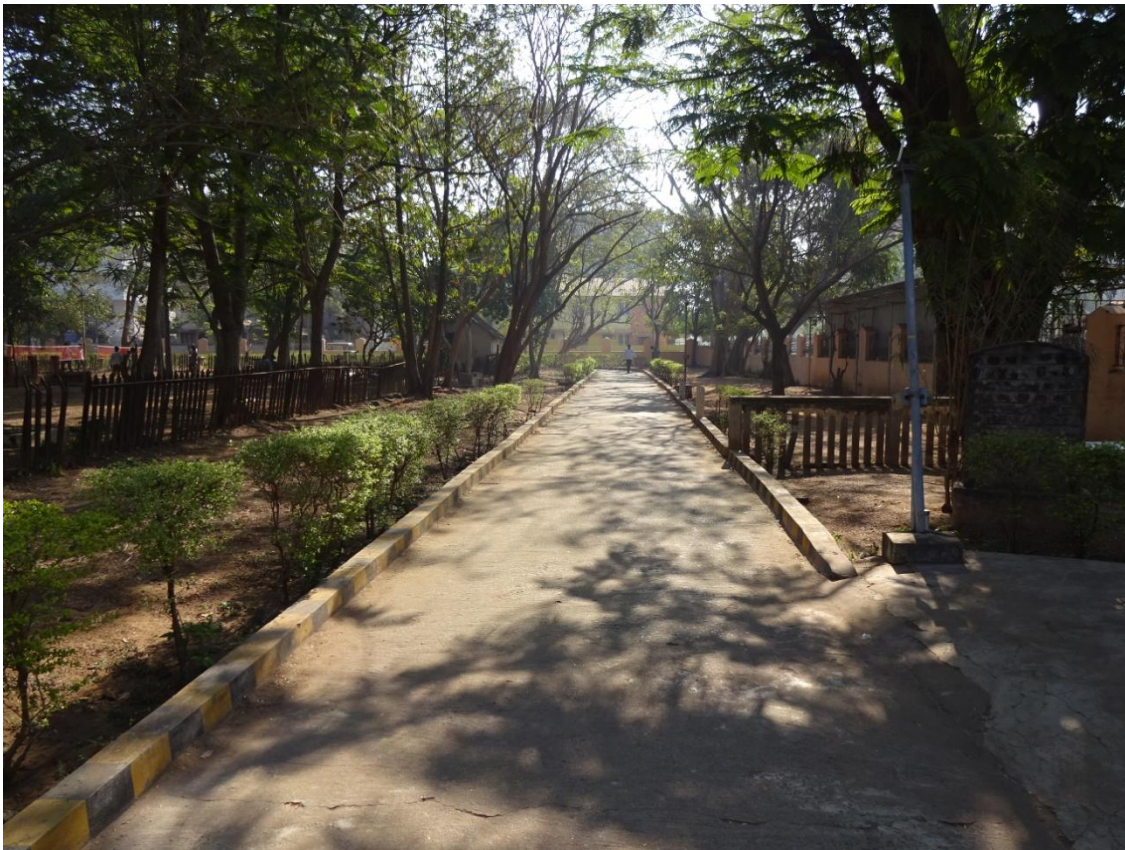
Existing Pathway condition
